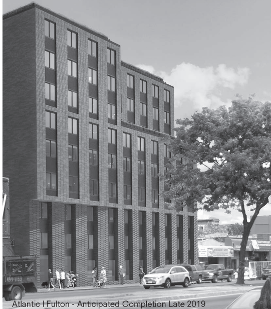
Atlantic | Fulton - Anticipated Completion Late 2019
