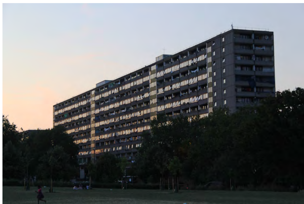
■ View of the estate from Burgess Park
