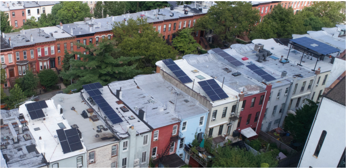
(Above) Neighbors in Park Slope organized a group solar purchasing project with Brooklyn SolarWorks. The solar installations depicted are coordinated around skylights and mechanical equipment and cover only a portion of the residential roofs. On the far right, a raised solar trellis allows access across the whole roof. Photo credit: Misbrenner, Kelsey, et al. "Solar and the City: Creative Solutions Can Grow Solar in NYC." Solar Power World, 11 Feb. 2021.
