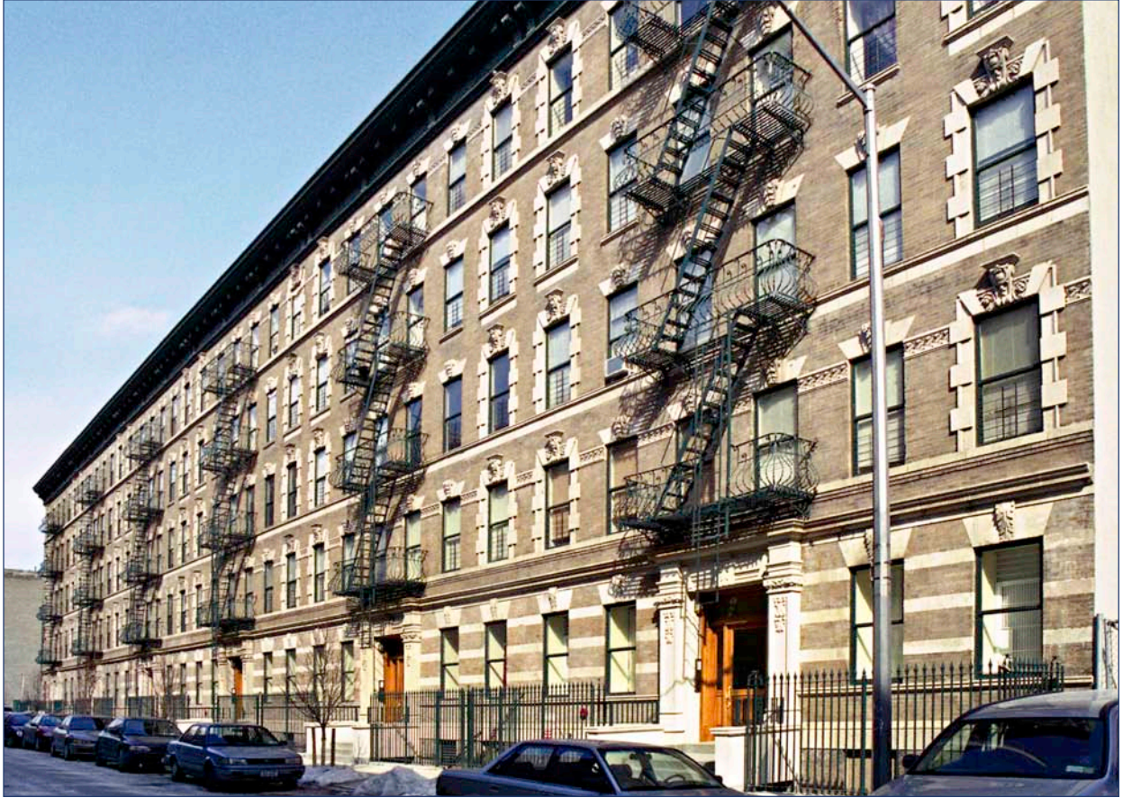
The same property following city financed rehabilitation. Photo © L. Racioppo, HPD/NYC
