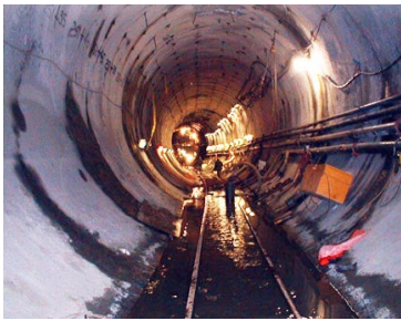
Third Water Tunnel
